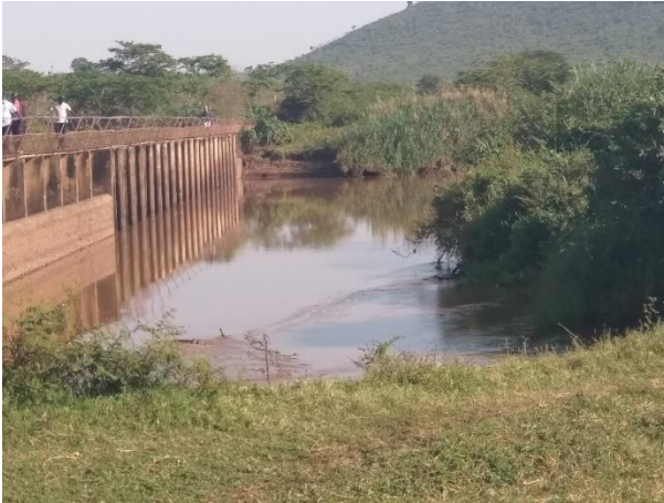
Picture: Gogo dam was visited by the survey team but was not sampled since it had receded back to the flowing river channel due to siltation.
