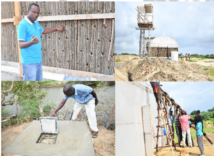
KMFRI AD Oceanography and Hydrography Dr Joseph Kamau explains how seawater greenhouse works. The Blue Economy pilot project at Kadzuhoni in Kilifi County will enable farmers in the semi-arid region to practise farming. The system extracts seawater from a borehole connected to the greenhouse, converts the water into vapour, and utilizes the cooling and humidifying power of vapour produced from evaporating salt water. The condensed water is then collected in a water tank and used for farming. In this project, Dr Kamau was assisted by KMFRI Engineers Dickson Aloyo and Joselyn Kendi | Photos by Jane Kiguta
