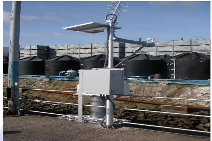
Mombasa sea level monitoring station
