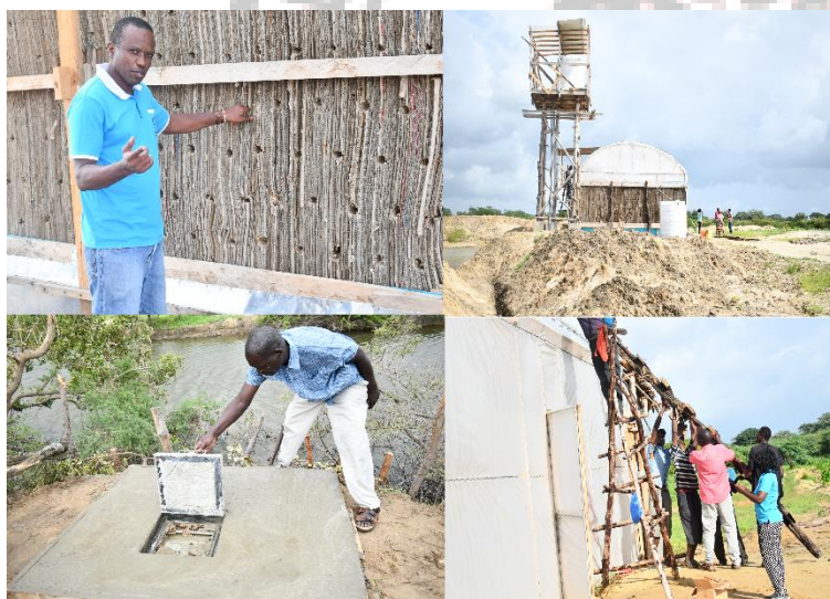
KMFRI AD Oceanography and Hydrography Dr Joseph Kamau explains how seawater greenhouse works. The Blue Economy pilot project at Kadzuhoni in Kilifi County will enable farmers in the semi-arid region to practise farming. The system extracts seawater from a borehole connected to the greenhouse, converts the water into vapour, and utilizes the cooling and humidifying power of vapour produced from evaporating salt water. The condensed water is then collected in a water tank and used for farming. In this project, Dr Kamau was assisted by KMFRI Engineers Dickson Aloyo and Joselyn Kendi | Photos by Jane Kiguta
