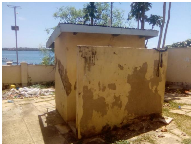
Plate 4-12; Pit latrine at Fisheries office Shimoni
