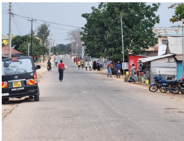
Plate 4-6: Tarmac Road Connecting Shimoni Market to Ramisi-Lunga Lunga highway at Kidimu
