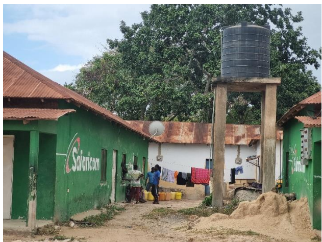
Plate 4-10: Water Pump to storage from a shallow well at Shimoni Market.
