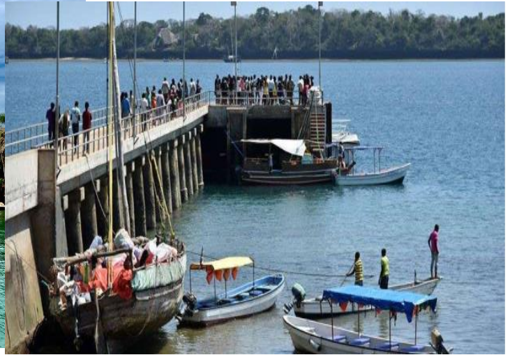
4D: Refurbished KeFS-jetty for loading and offloading for tourist visits
